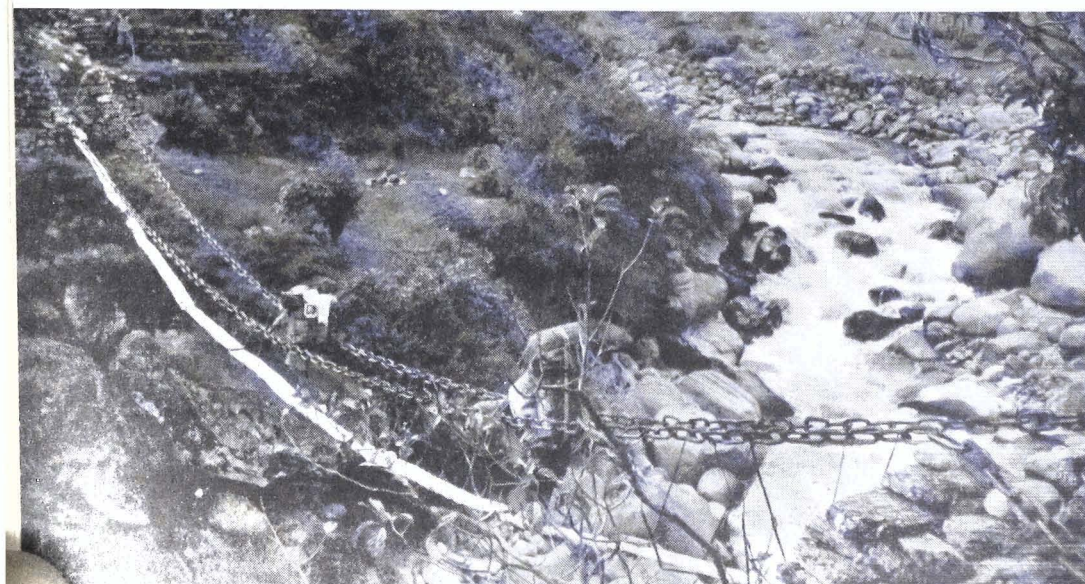
One of the safer bridges on the route from Kathmandu. The stout chains were forged at Those
